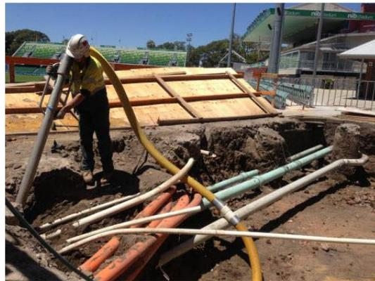
TerraVac's vacuum excavators are a **unique and versatile** self-contained unit which utilise a **powerful vacuum system** in combination with **regulated high pressure water** lance fitted with a
